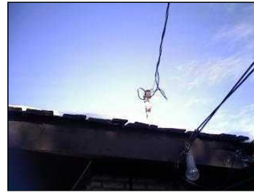
Reference photo. View of weatherhead.
